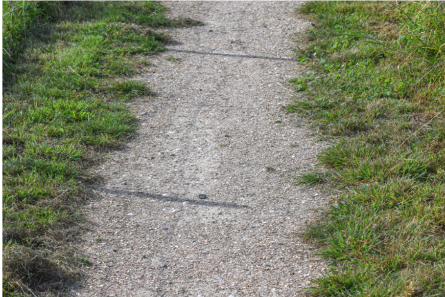
Halfverharde smalle parkpaden
